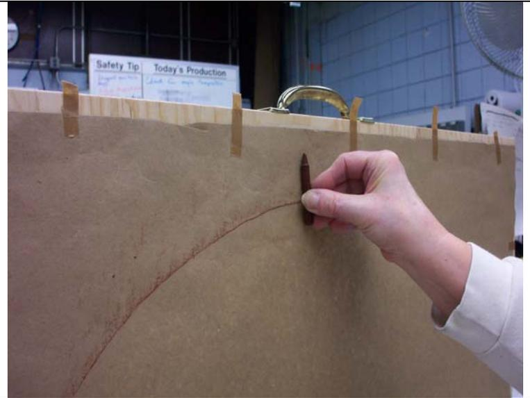
2. Being careful not to press against the template paper while tracing, draw an exact outline of the window opening. Pressing on the template paper may distort the paper and cause the wrong size to be made.
